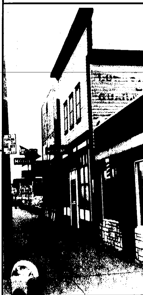
Looking south on 101 Street in 1961. Photo from the City of Edmonton
